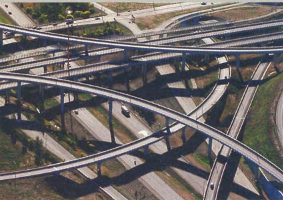
TANGLED WEB Western Sydney's ever-expanding maze of freeways, arterial roads and overpasses bodes ill for the looming energy crisis
